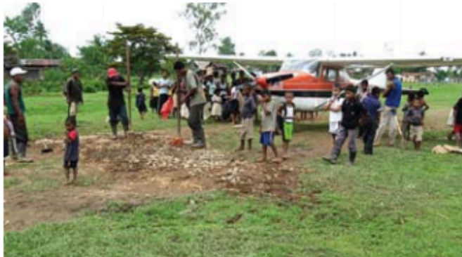
Repairing a muddy runway.
